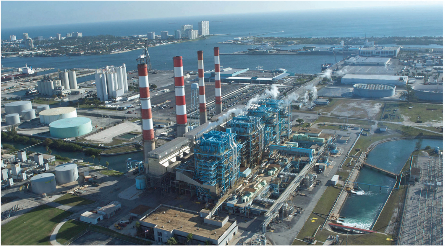
Port Everglades Plant Hollywood, FL
